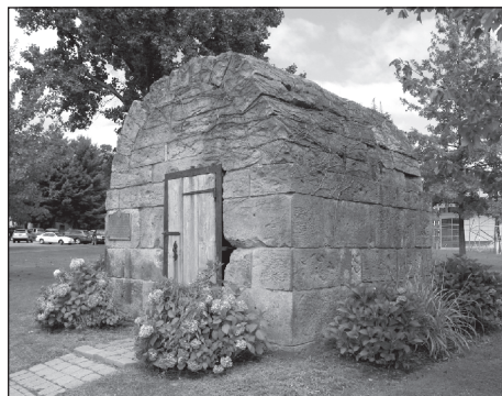
Above is the Holland Land Company vault in Mayville, N.Y. The company required that all of its records be stored in a bank vault, or a vault of its own.
